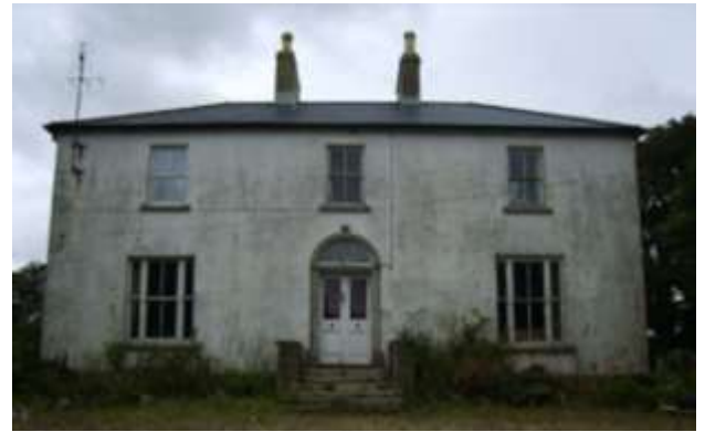
Rathmacknee Rectory. Source Department of Arts and Heritage Ireland
