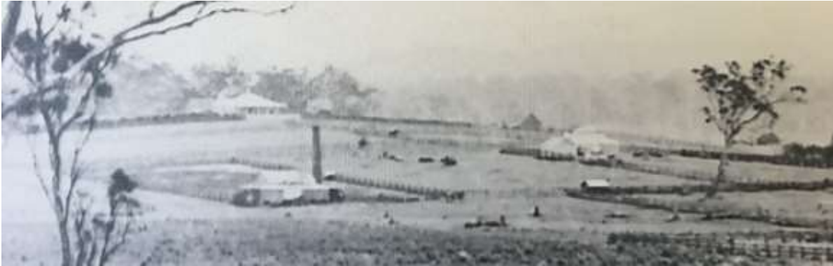
“West End” appears in this old photo just above and to the left of the chimney stack of the flour mill in Shore Street. Photo taken from Police sergeant’s residence in Page Street -photo of it put onto canvas, Marie Traynor
