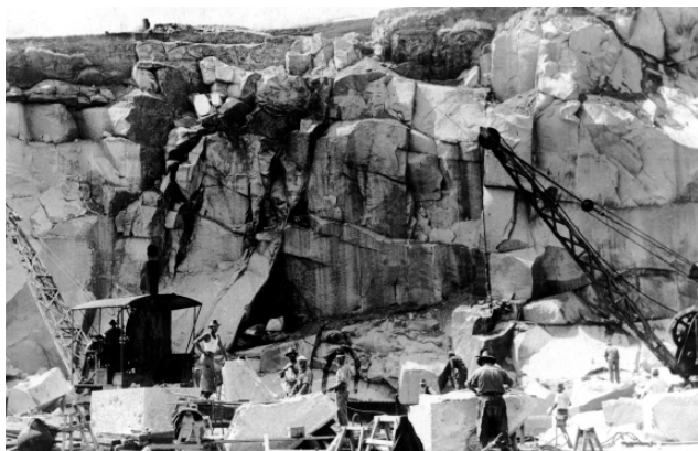
Above: Work at the Quarry Face
