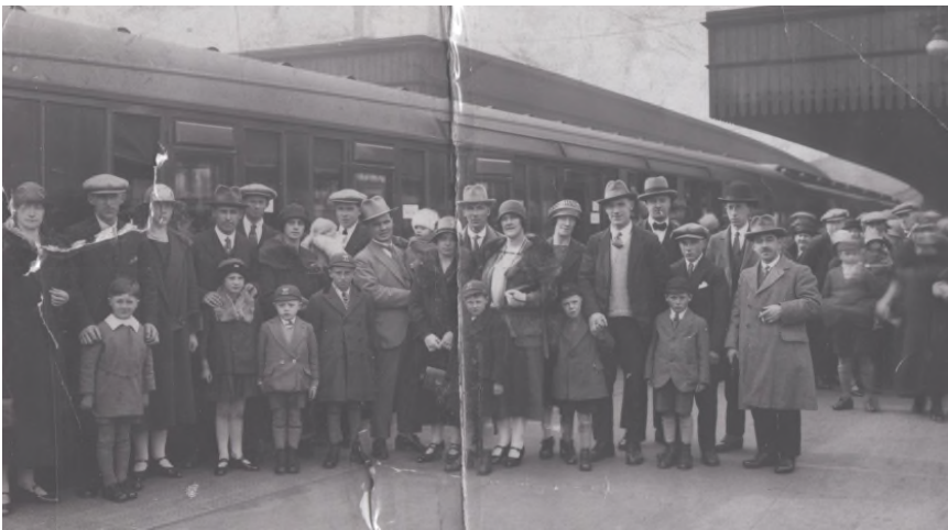
Above: The Pakeha group at Aberdeen Joint Station March 1926.
