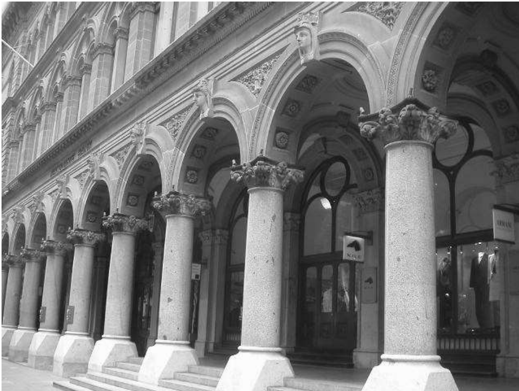
Columns of GPO, Louttit Quarry granite.
